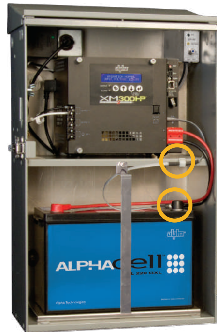
Fig. 1-8, Temperature Probe Locations
