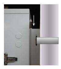
3. Securely fasten the enclosure to the bracket using the six 5/16" bolts, lock washers and fender washers (supplied).
