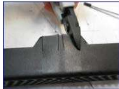
Cut holes to allow cable access
